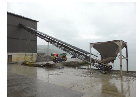
- Hardanger betong as
